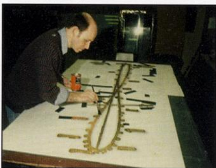
Figure 12: Work on the glass panel - on the left the stencil is being applied before shot blasting; on the right the gold leaf is being given a protective lacquer.
